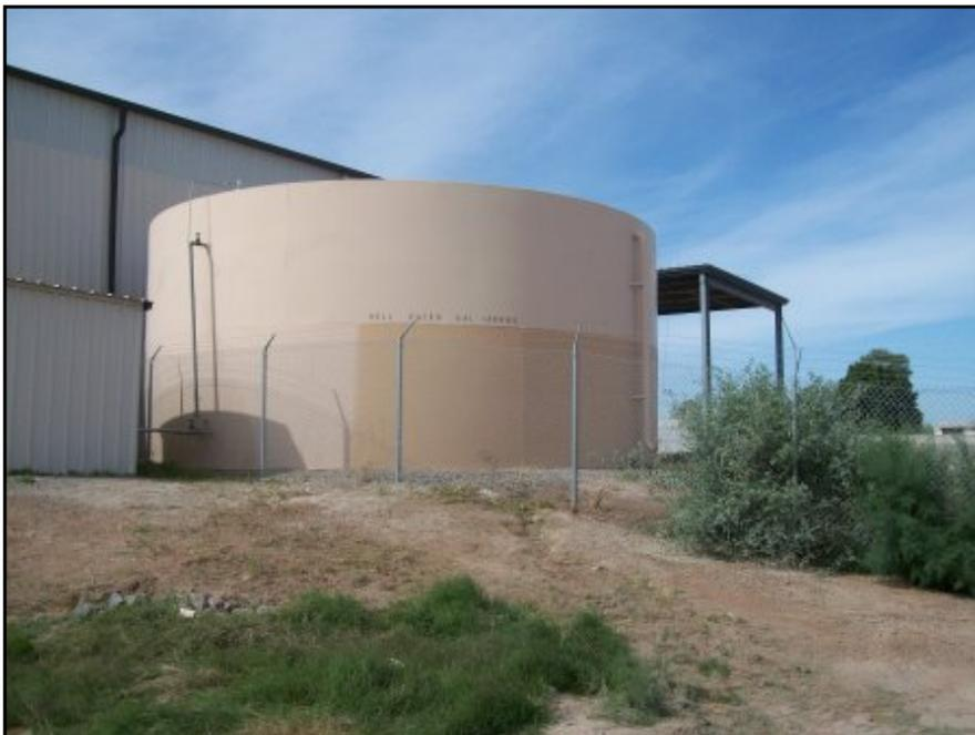
120,000-gallon water storage tank and associated pumphouse located on the northwestern portion of the site.
