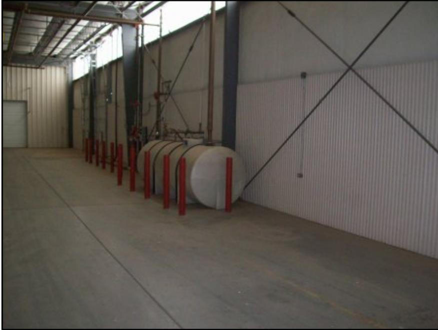
1,000 gallon water tank used for the evaporative cooling system.
